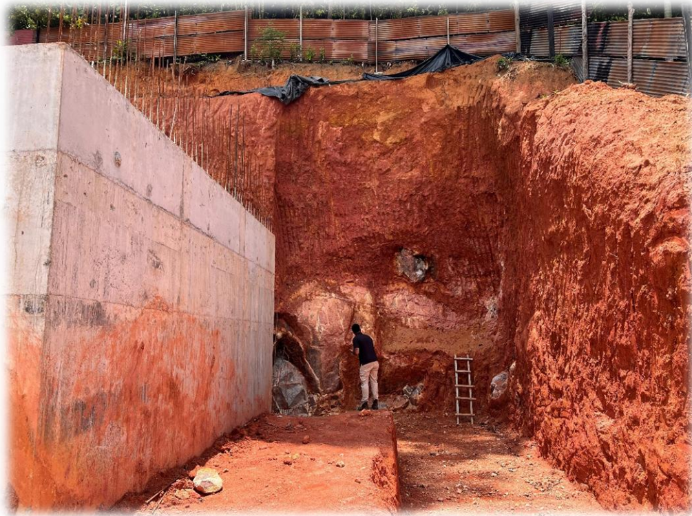
Figure 25-PA engineer on site inspection
