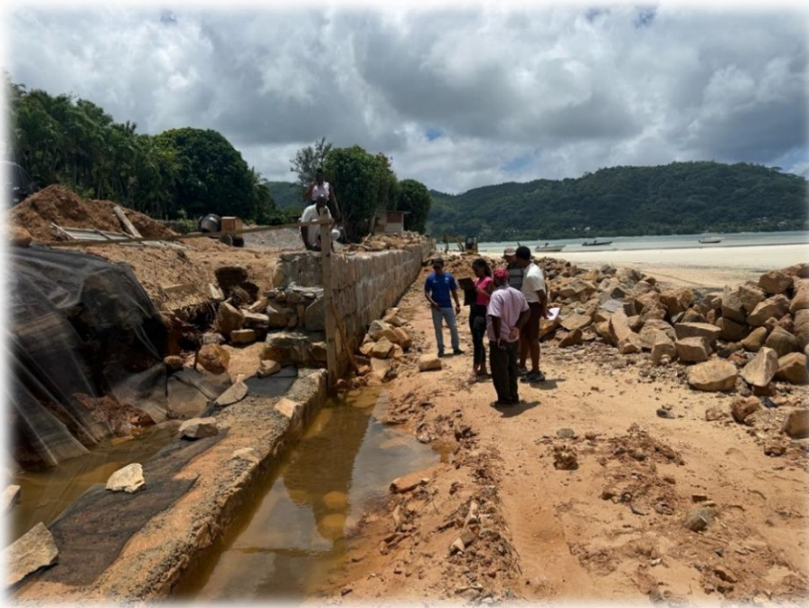
Figure 23 –The Quality Assurance & Building Control unit on site inspection.
